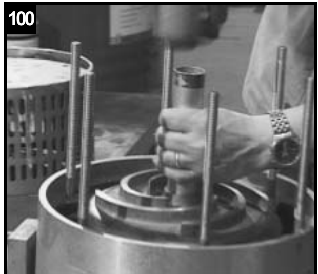
100 Tap split bushing into position.
