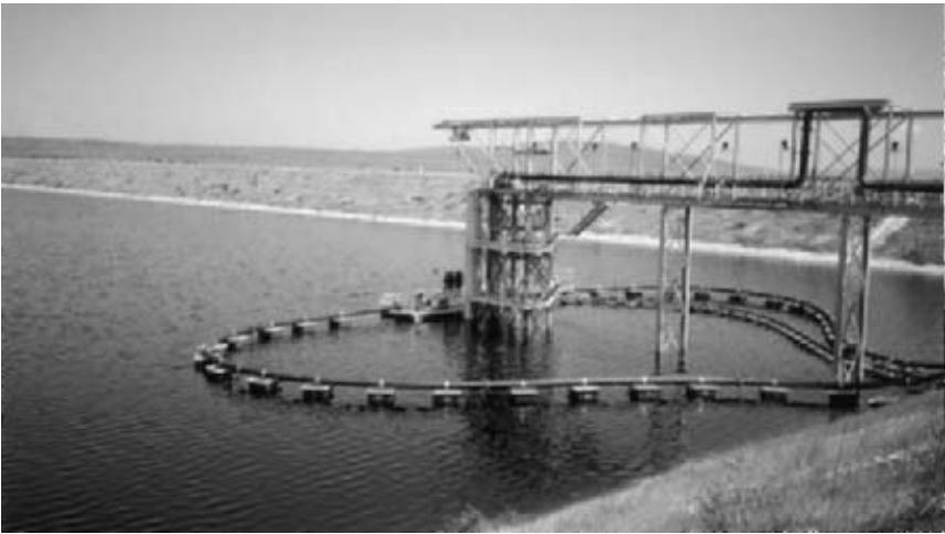
FIGURE 6 Float-mounted pumps designed to skim the clean liquid in a settling pond (Hazleton Pumps, Inc.)
