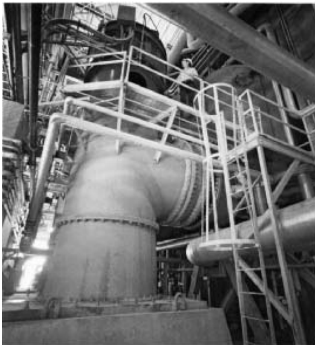
FIGURE 112 Vertical propeller pump installed (Flowsolve Corporation)
