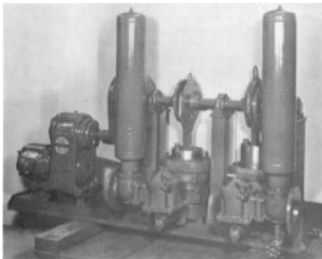
FIGURE 9 Plunger-type sludge pump (ITT Marlow Pumps)
