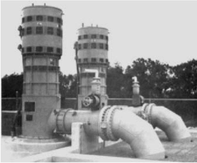
FIGURE 10 Raw water pumping station for North Texas Municipal Water District, showing vertical turbine pumps with variable-speed drives (Flowserve Corporation)
